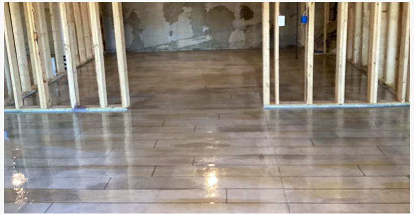
Residential barn with concrete wood floor overlay.
