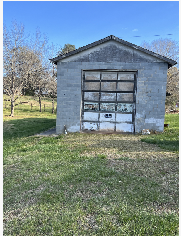
Before new garage door has been installed
