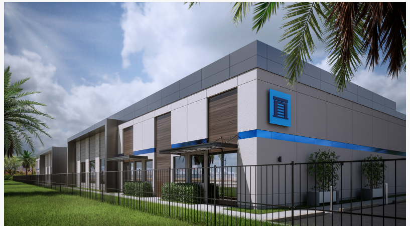
Luxury Warehouse Development Lakeland FL
