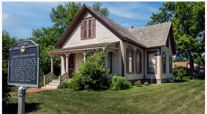
The Willa Cather Childhood Home, a National Historic Landmark, is undergoing an extensive restoration during the author's 150th birthday year. It will reopen later in 2023.
