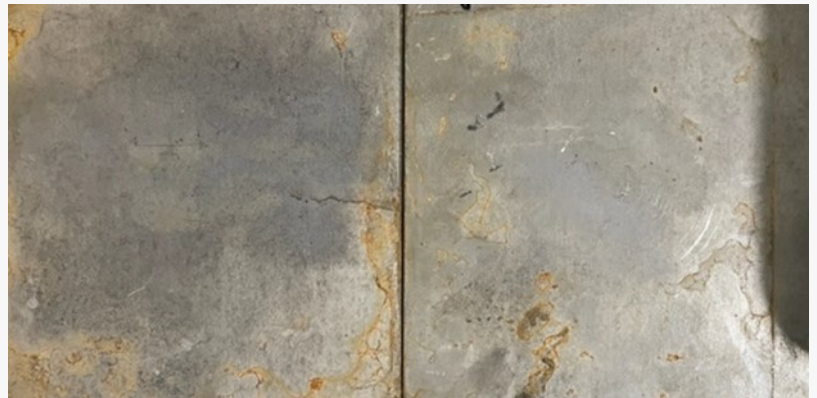
Pre blasted steel
