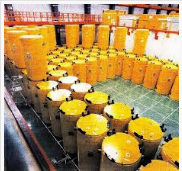
Graphite spent fuel storage casks at Juelich.
