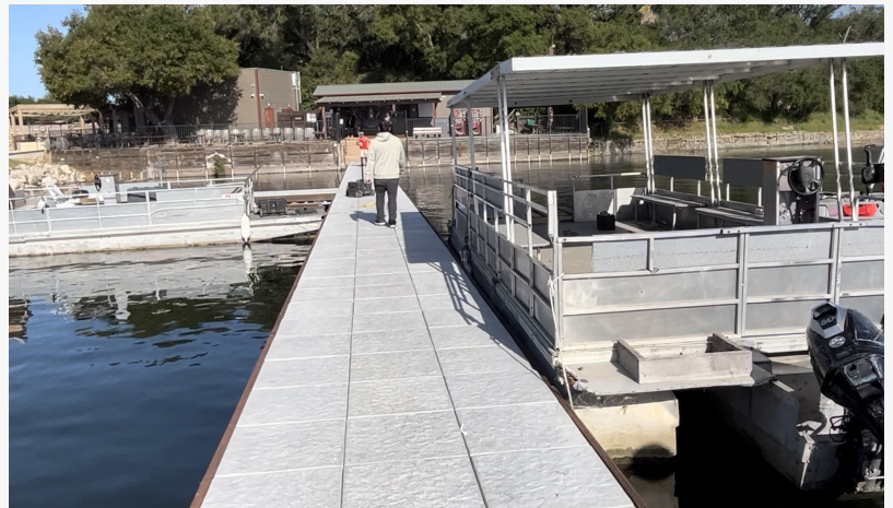
The new impressive dock built by hospitality company, ExplorUS.
