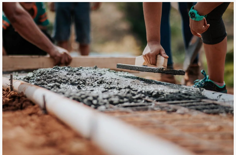
Remove Concrete from Bricks
