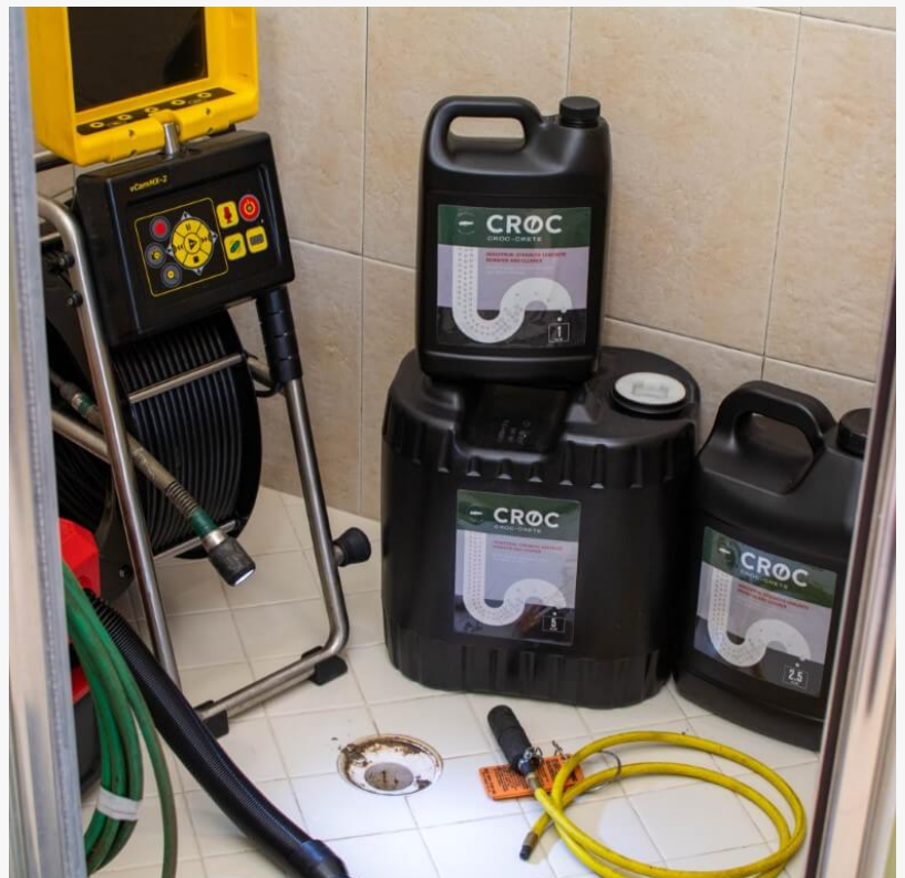
Remove Concrete from Plumbing
