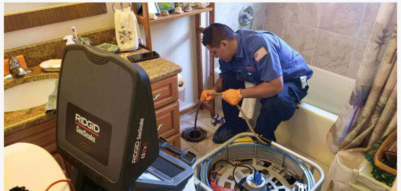
Solution to Remove Concrete from Plumbing
