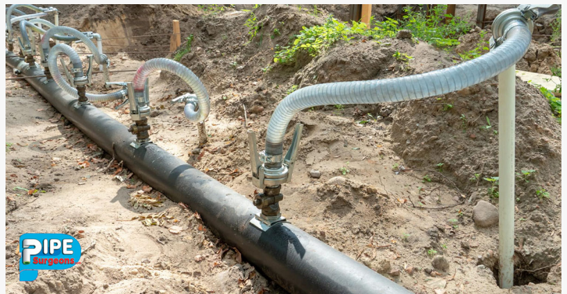
Pipe Repair Service in Port Saint Lucie
