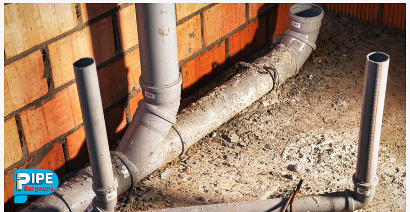
Trenchless Pipe Repair Services Port Saint Lucie
