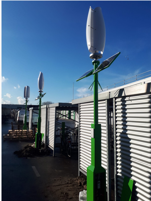
Wind and Solar E-bike Charging Poles
