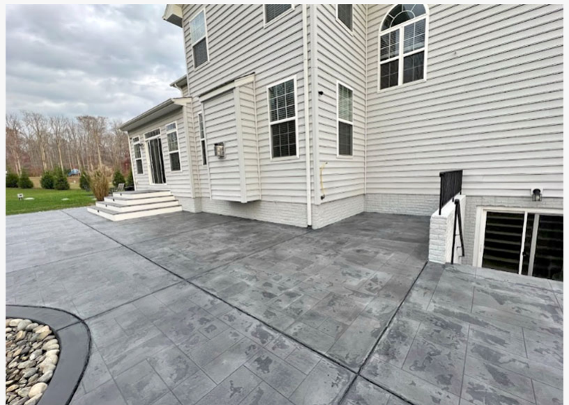
Tuscan slate stained concrete patio installed by LNS Concrete.
