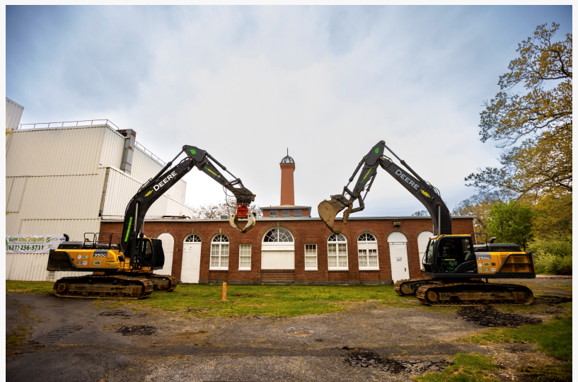
This photo shows the Wardenclyffe laboratory of Nikola Tesla alongside demolition equipment that will be used to remove non-historical buildings surrounding the lab.
