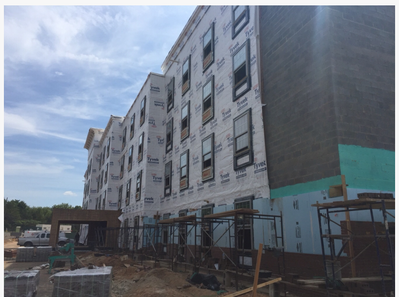
This is the construction site where the mason was injured
