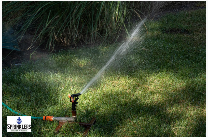
Irrigation Sprinkler Repair in Dallas
