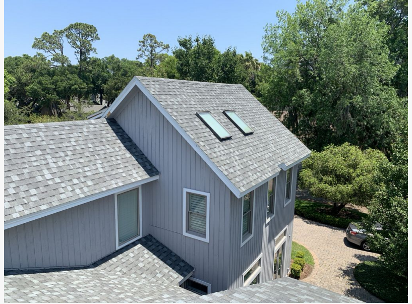
roof leak repair in Jacksonville
