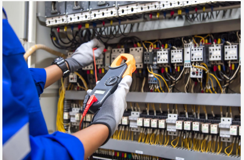
Experienced Electrician Port St. Lucie
