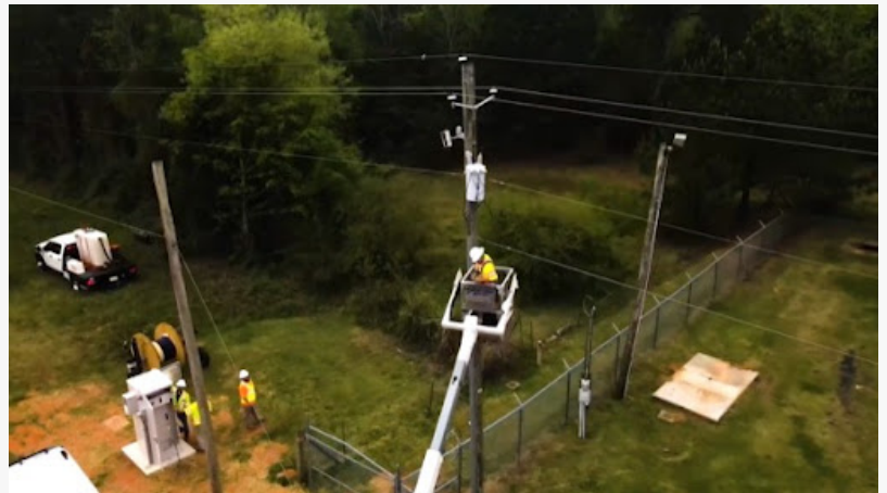
Engineers attaching networking equipment to telephone poles
