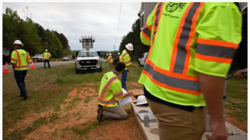
Engineers from Point Broadband lay fiber in Macon County, Alabama
