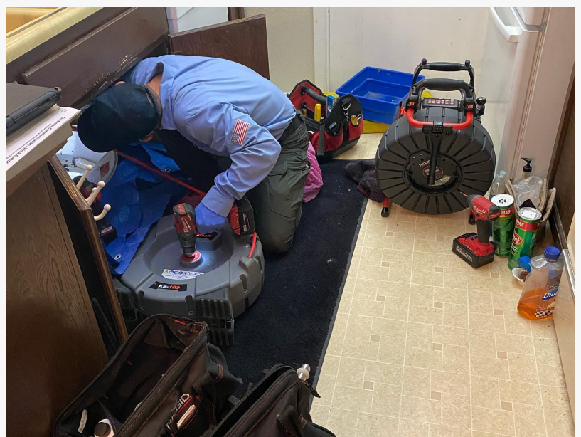
gilbert drain cleaning plumber
