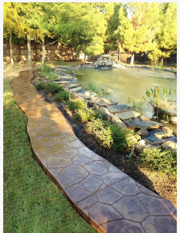
We poured this beautiful stamped concrete walkway for a customer.
