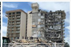
The partial collapsed of the Florida Champlain Towers South, showed not all that different to buildings nearby. That is, it is difficult to inspect and predict when the disaster will happen for a concrete buildings that had concrete overly weakened and rebar corroded.
