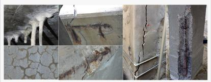
These pictures are examples of several forms of concrete weakening and rebar corrosion. These concrete chemical reactions and rebar corrosion weakened the structure internally with little exterior damages. To assess the damage for remedial actions are not so obvious.
