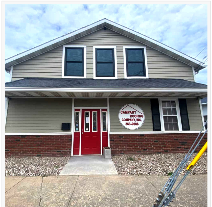
Campany Roofing in Oneida NY
