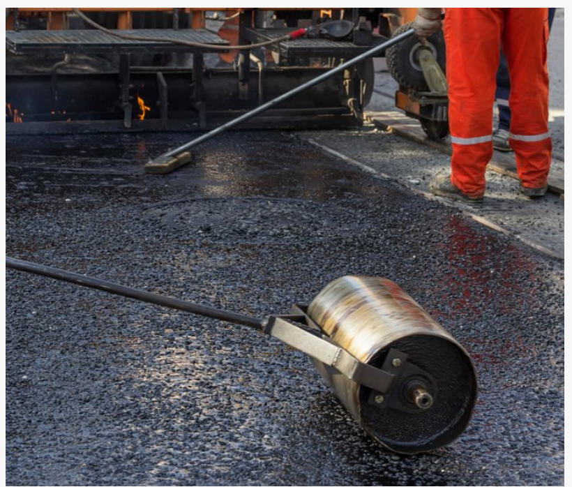
paving and seal coating for Arlington homeowner
