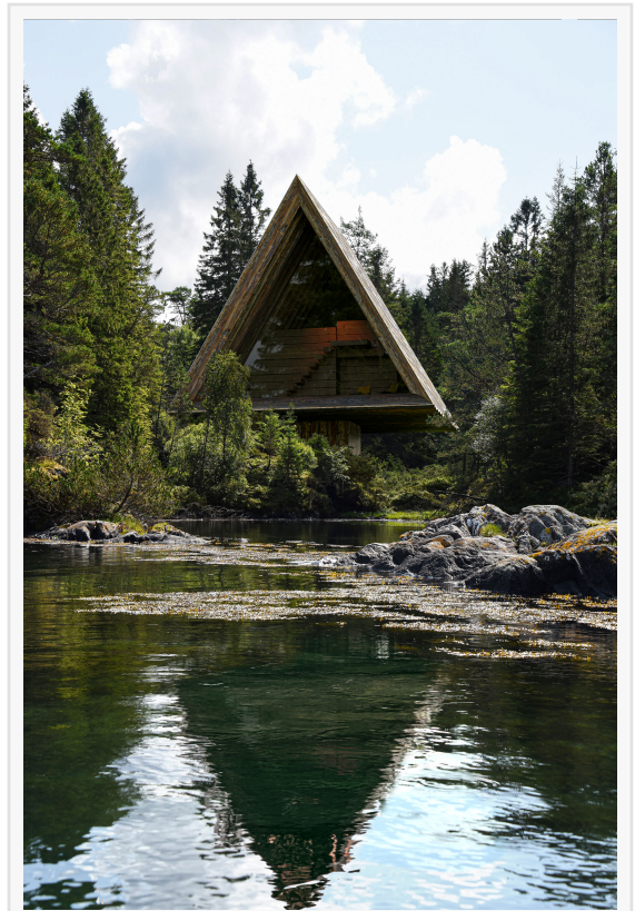
Wood house, a self contained house on the east shore of the island. The design has two bedrooms, a kitchen & a living area looking out through a vast 8m triangular vista.
