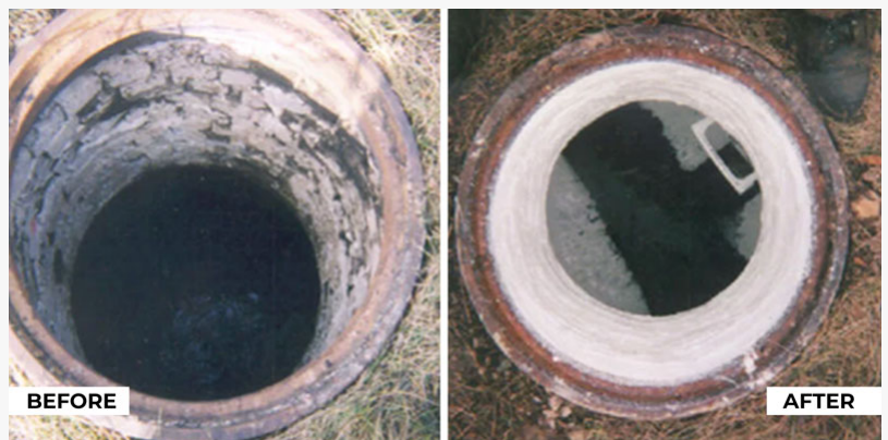
Before and after of manhole sealing
