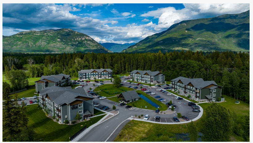
The Highline Apartments - Columbia Falls, Montana
