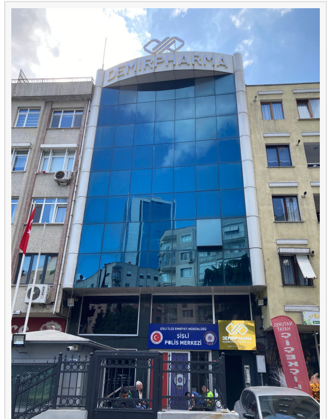
Demir Pharma Head Office
