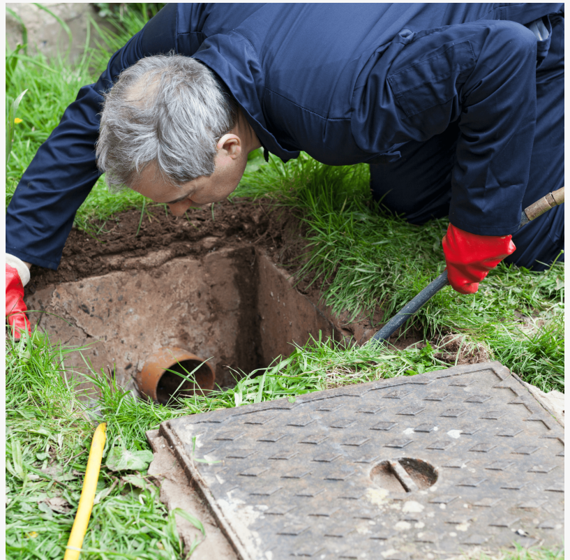
The drain must first be inspected before installing drain lining.
