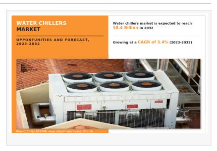
Water chillers are the type of refrigeration systems that use water as the secondary refrigerant. Such systems are used for more complex and larger HVACR (heating, ventilating, air conditioning, and refrigeration) applications. These chillers help in lowering the temperature of water. A water chiller makes use of the heat exchanger in order to cool down the fluid.
