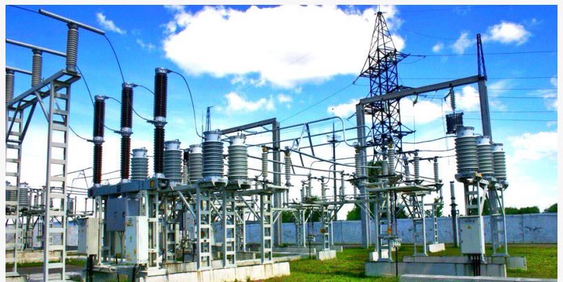
High Voltage Equipment Market
