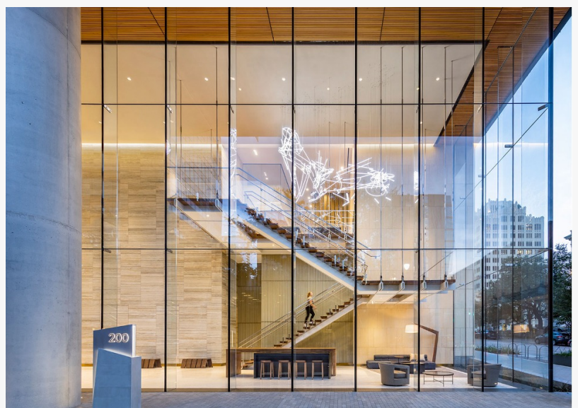
Sentech Architectural Systems and Faour Glass Technologies' Slimpact product line expand the range of tested impact-resistant structural glass systems.
