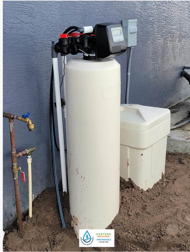
Water Treatment System Installation in Port St. Lucie
