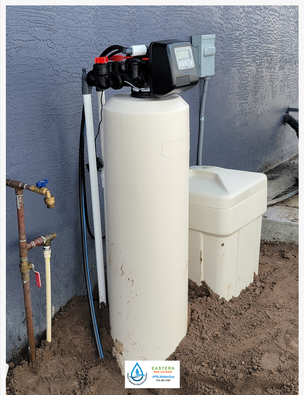
Water Softener System Installation Port St. Lucie
