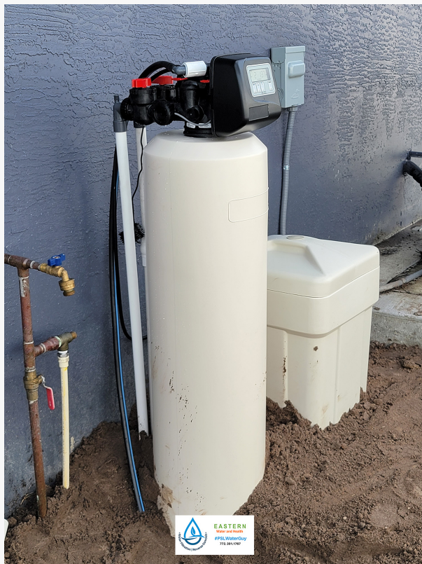
Water Softener System Installation Company
