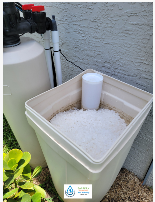
Water Treatment System Installation in Port St. Lucie
