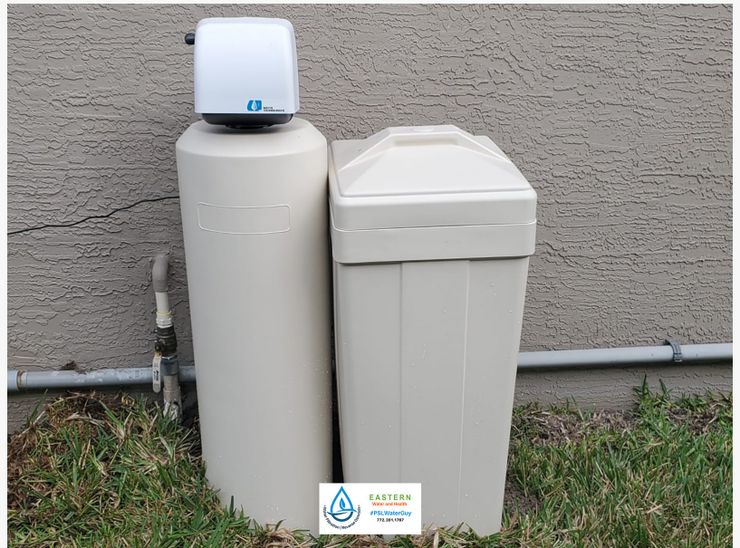
Water Softener System Installation Port St. Lucie
