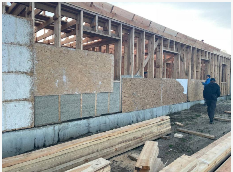
Detail showing hempcrete construction methods at Hemp Ukraine Recover construction site near Lviv, western Ukraine.
