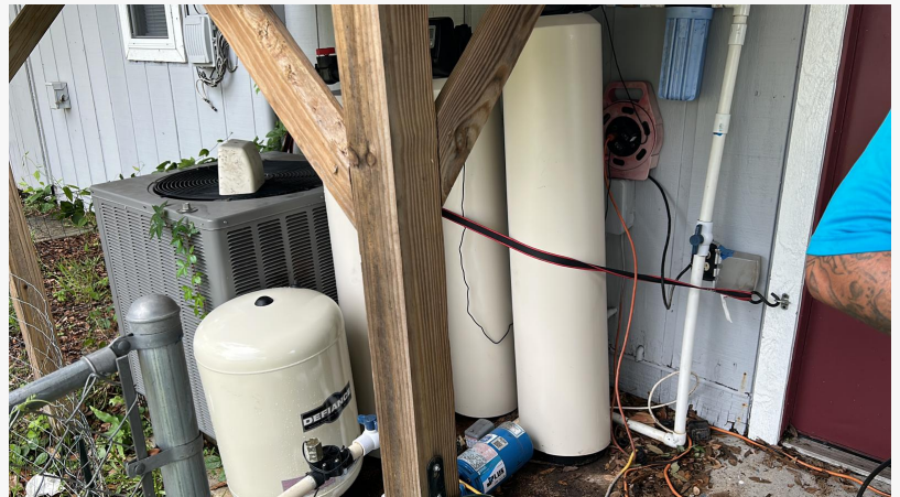
Well water treatment installation at a Lakewood Park residence
