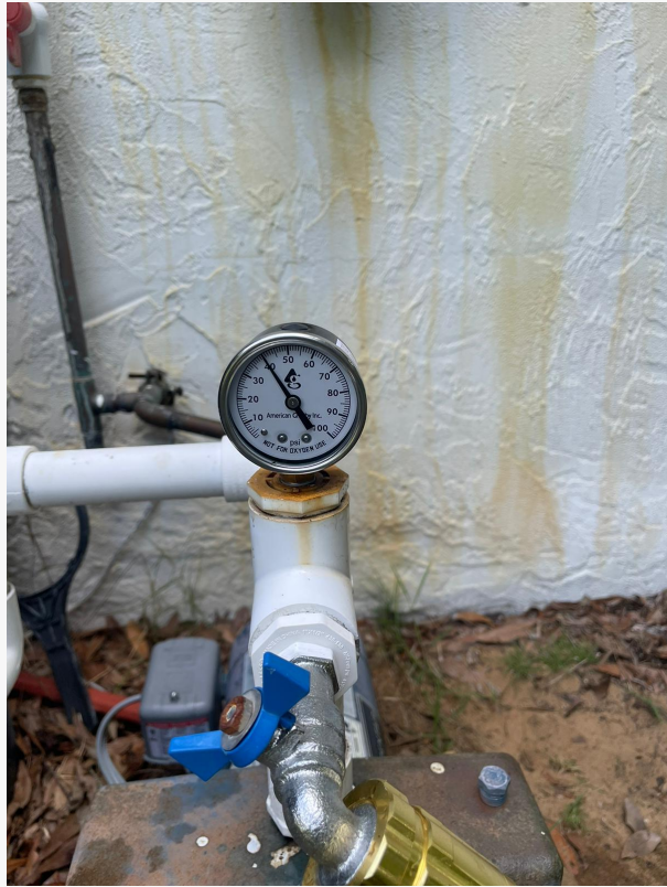
This pressure gauge was broken and needing replacement - Lakewood Park
