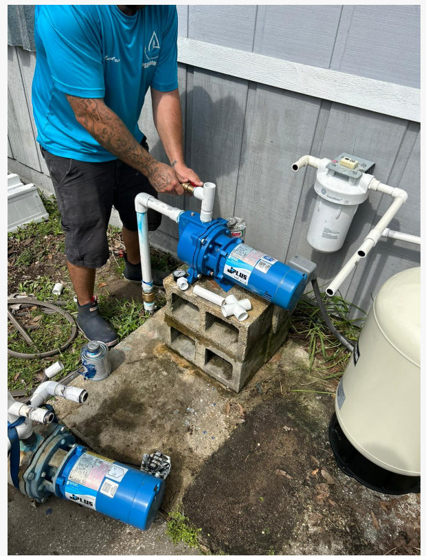
Lakewood Park well pump installation
