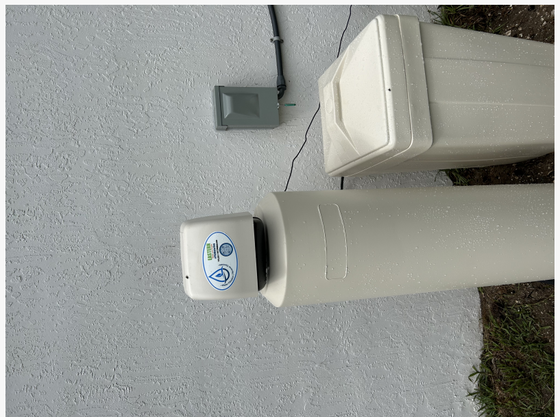
Port St Lucie Install of Water Softener
