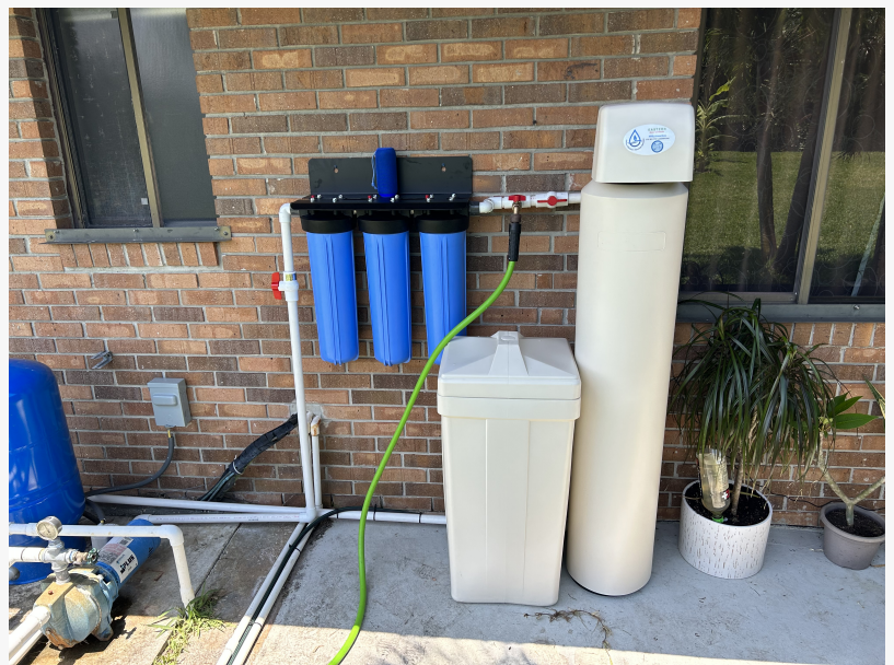
Installation of a Tank with A big John Sediment Filter
