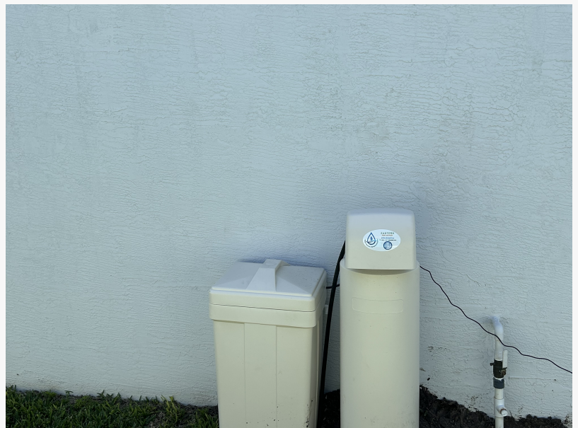
Salt Brine Tank with Softener
