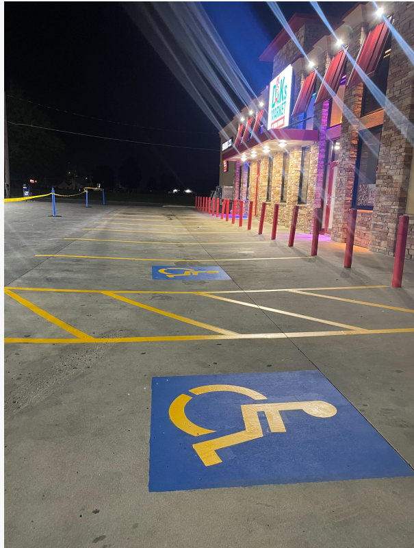
Parking lot striping job performed by Power Washing of Tulsa at Dak's Market
