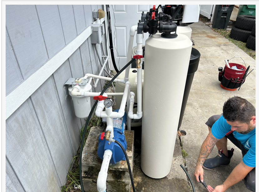
Pump swap out in Lakewood Park
