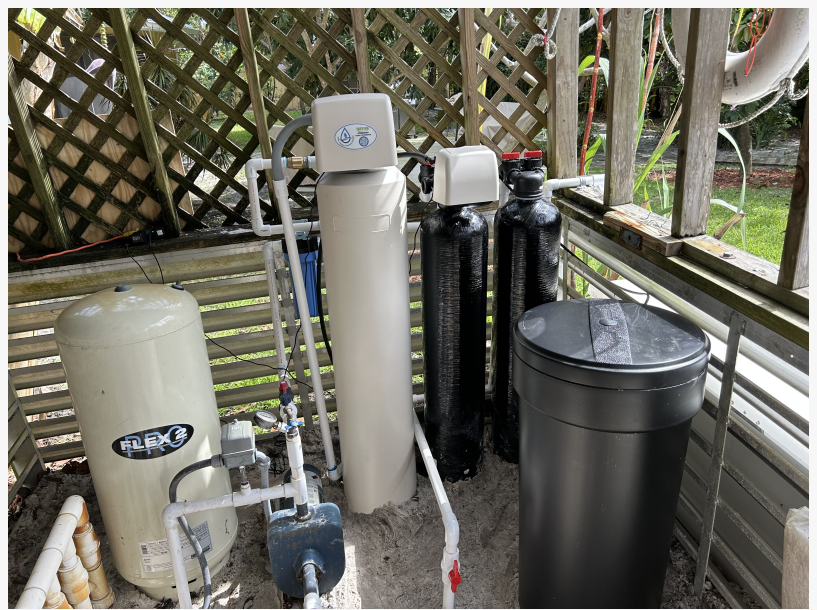
Well System Installed at Indian River
