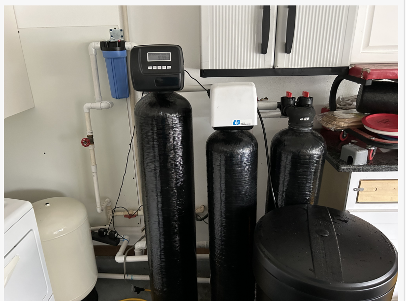
Installation of Triple Tank System
