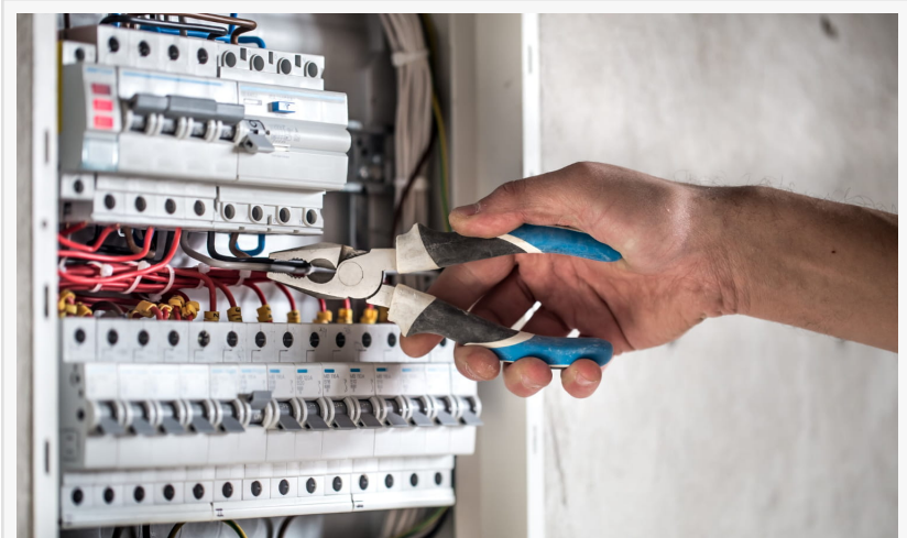
Generator Installation Service
