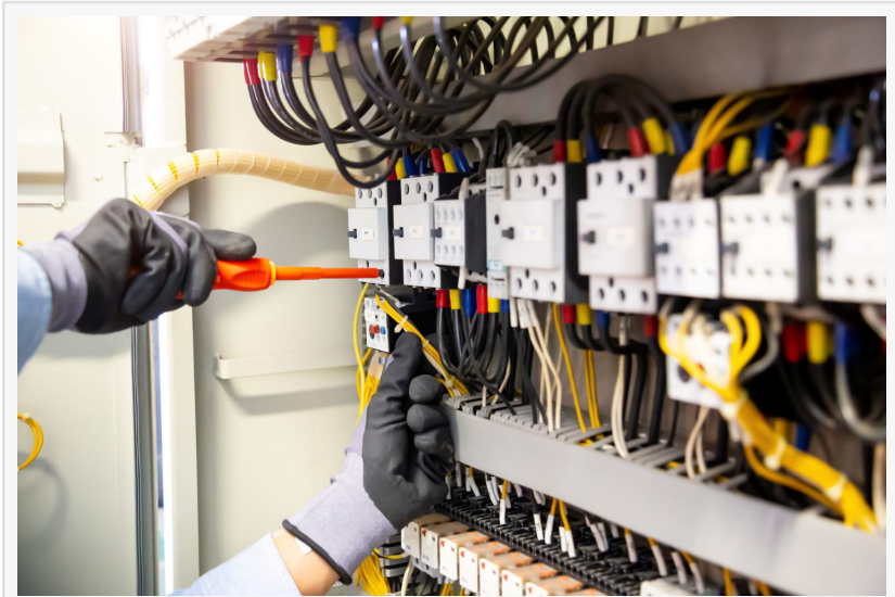
Commercial Generator Installation
