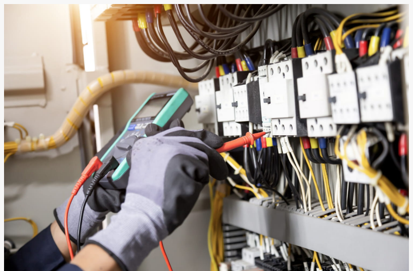
Generator Maintenance Service
