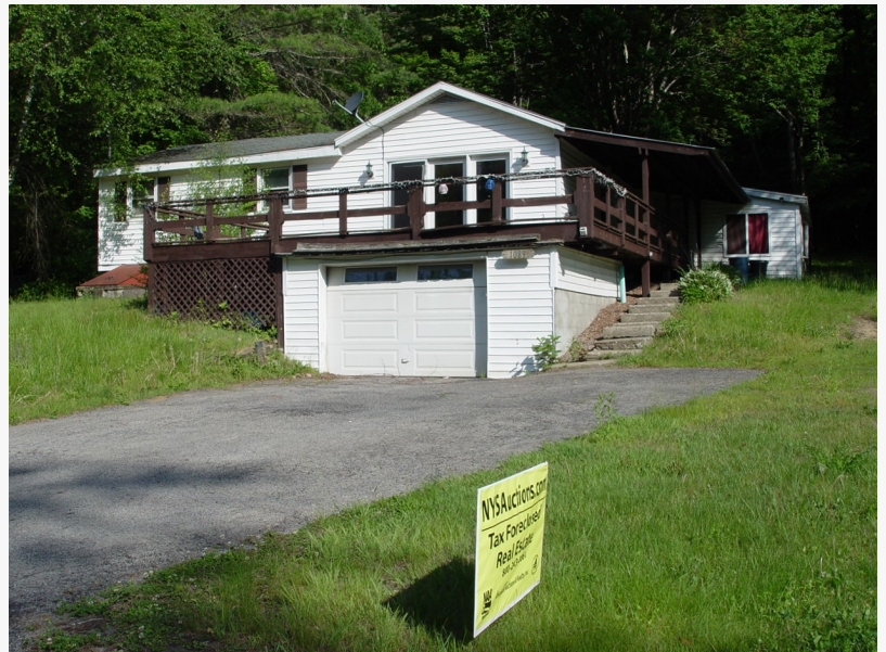
1089 County Hwy 123, Town of Northampton
