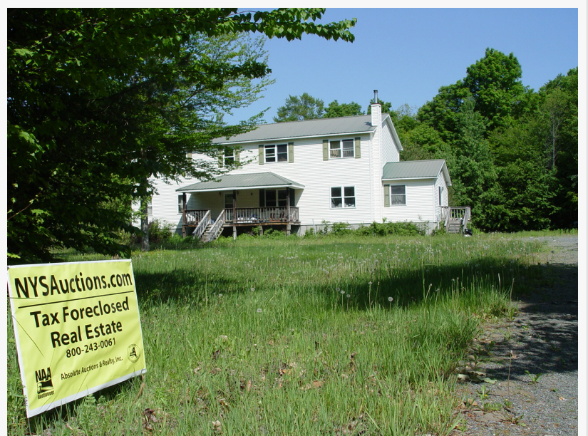
1162 Co Hwy 112, Town of Bleecker
