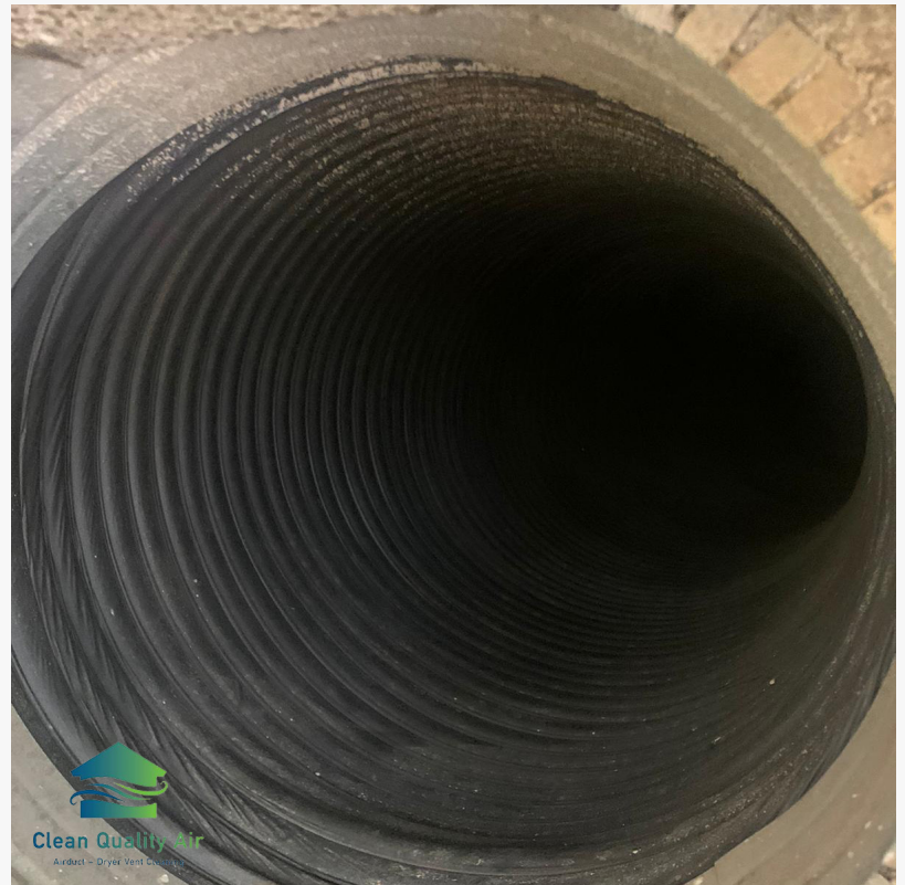
Air Duct Services
