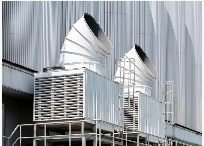
Air Duct Cleaning Services
