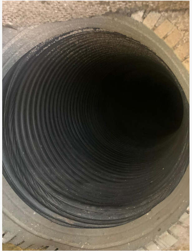
Fast and Reliable Air Duct Cleaning Port St Lucie, Air Duct Cleaning Port St Lucie
