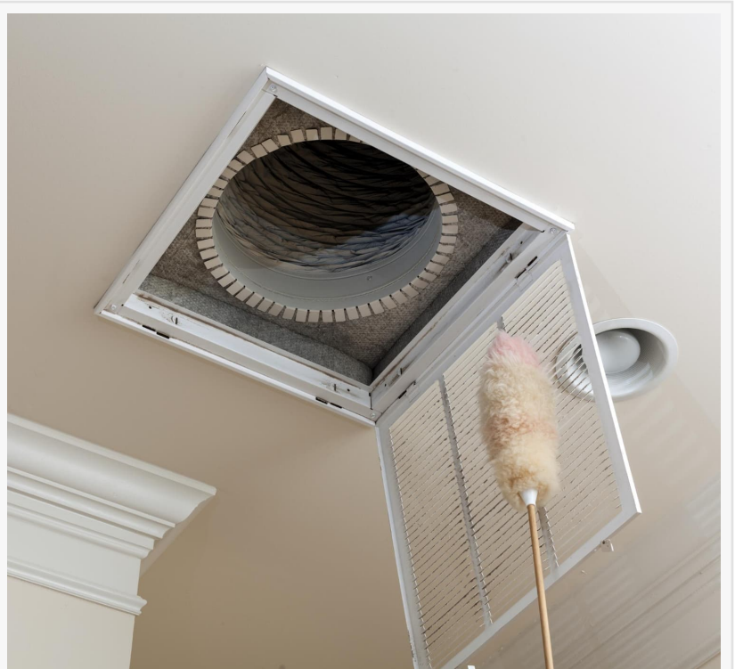
Air Duct Cleaning
