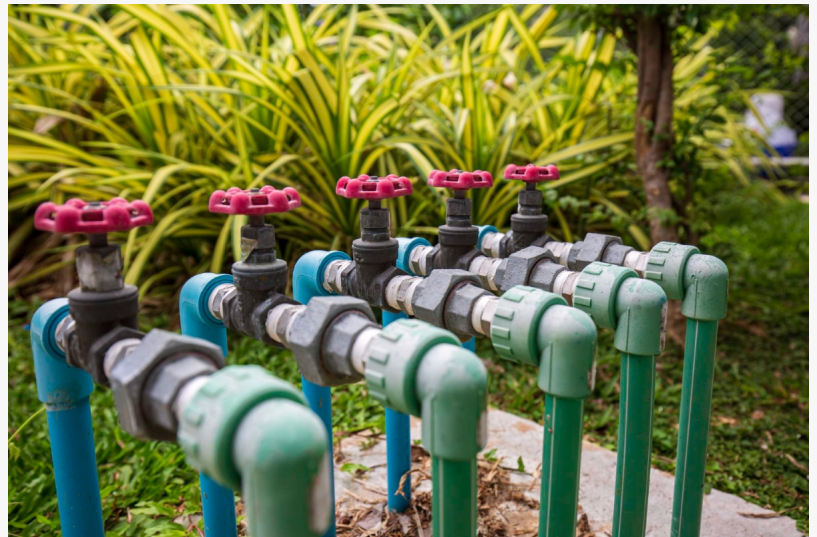
Pipe Relining Services
