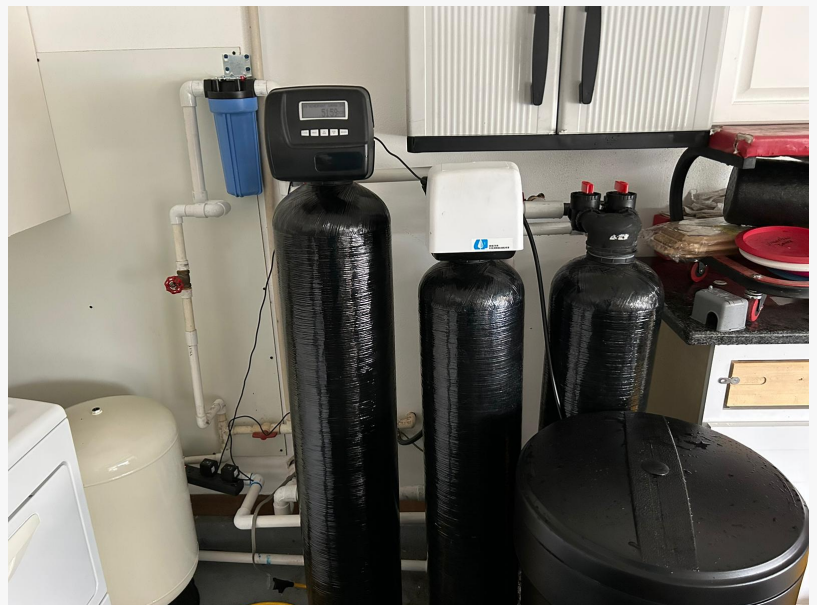
well water installation
