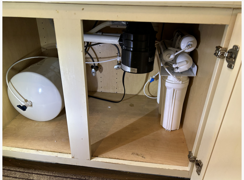
reverse osmosis install
