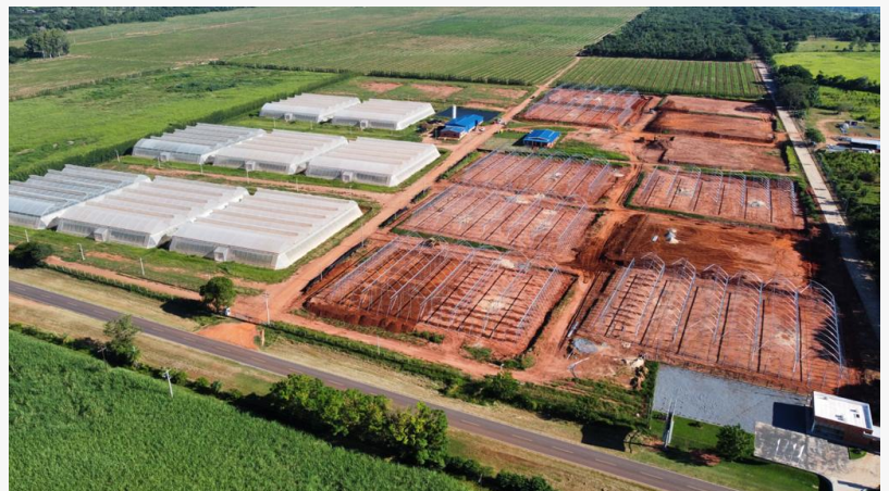
Greenhouses from Agri Terra Group
