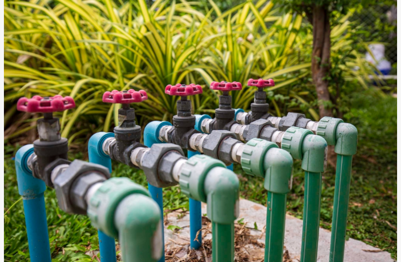
Pipe Relining Services
