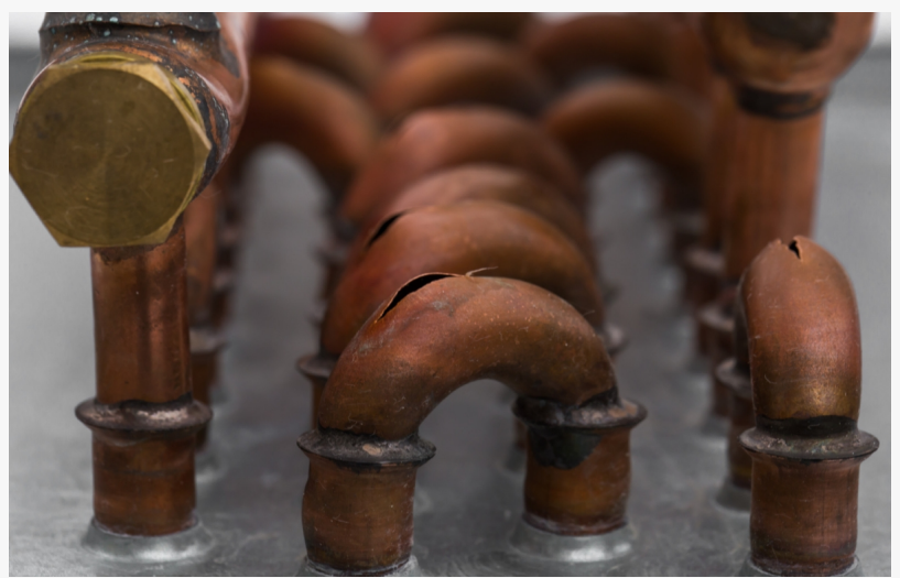
Pipe Relining Services
