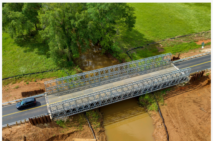
Acrow Detour Bridge in Texas
