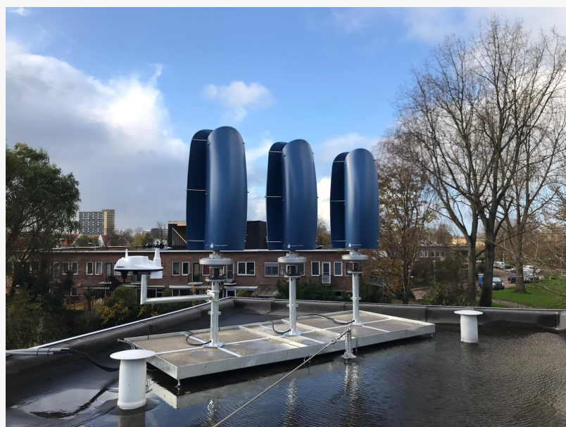
Flower Turbines Small Size Wind Tulip Installation
