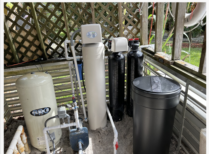
installation of pumphouse triple system
